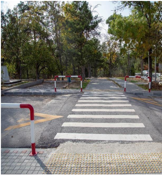
elevated pedestrian crosswalks
