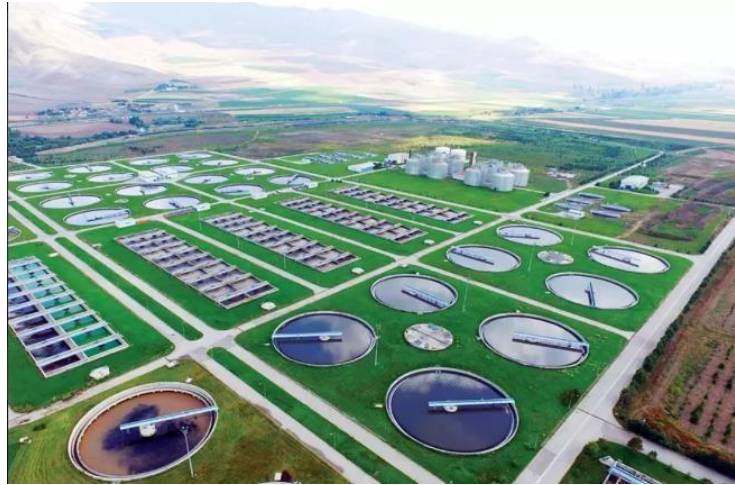
ASKİ, Conventional activated sludge process, Ankara ( http://www.aski.gov.tr/TR/ICERIK/Atiksu-Aritma/30 ).
