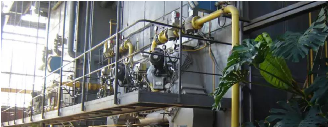
Eymir Pumping Station, processing drinkable water to be used in METU Campus
