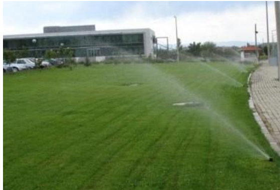
Recycled water used in irrigation
