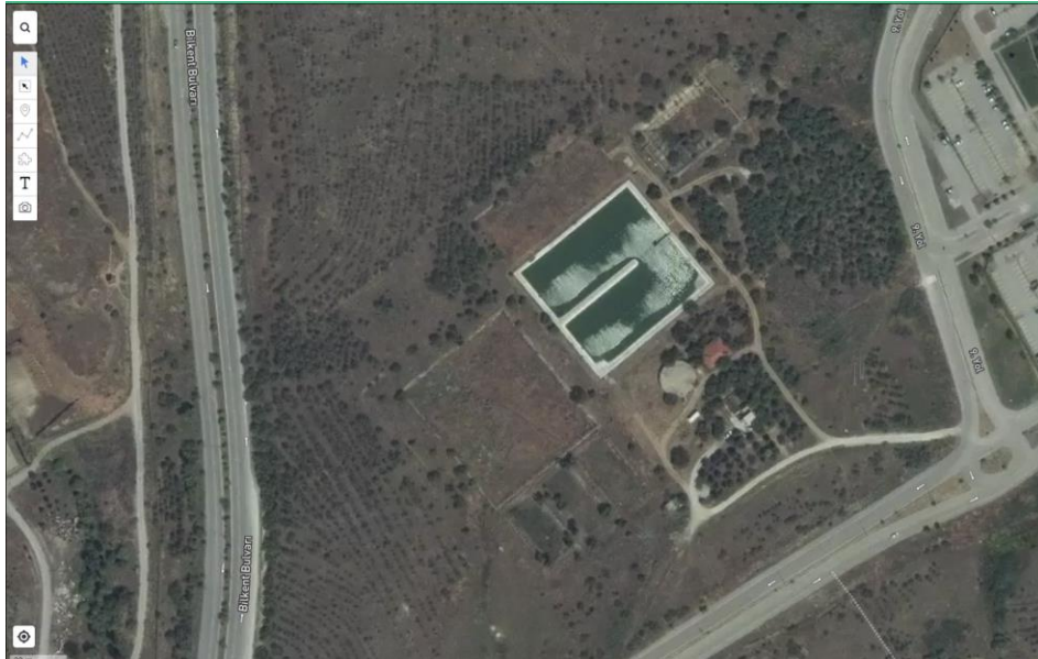
Water Recycling Plant (taken from Google Earth)
