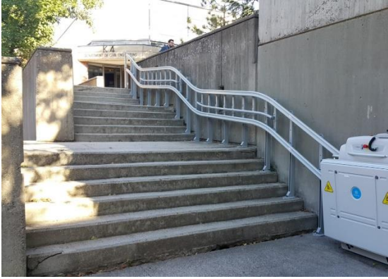
platform lifts for disabled
