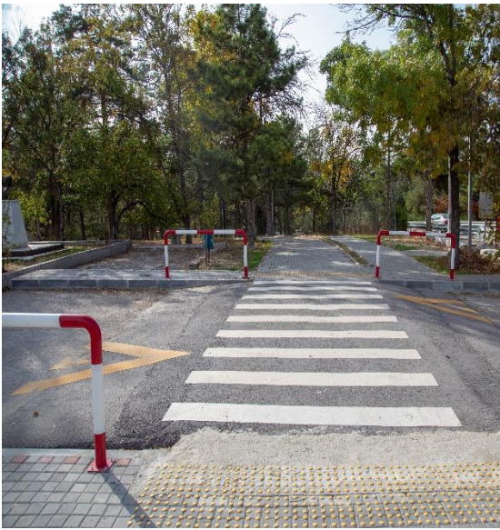
elevated pedestrian crosswalks
